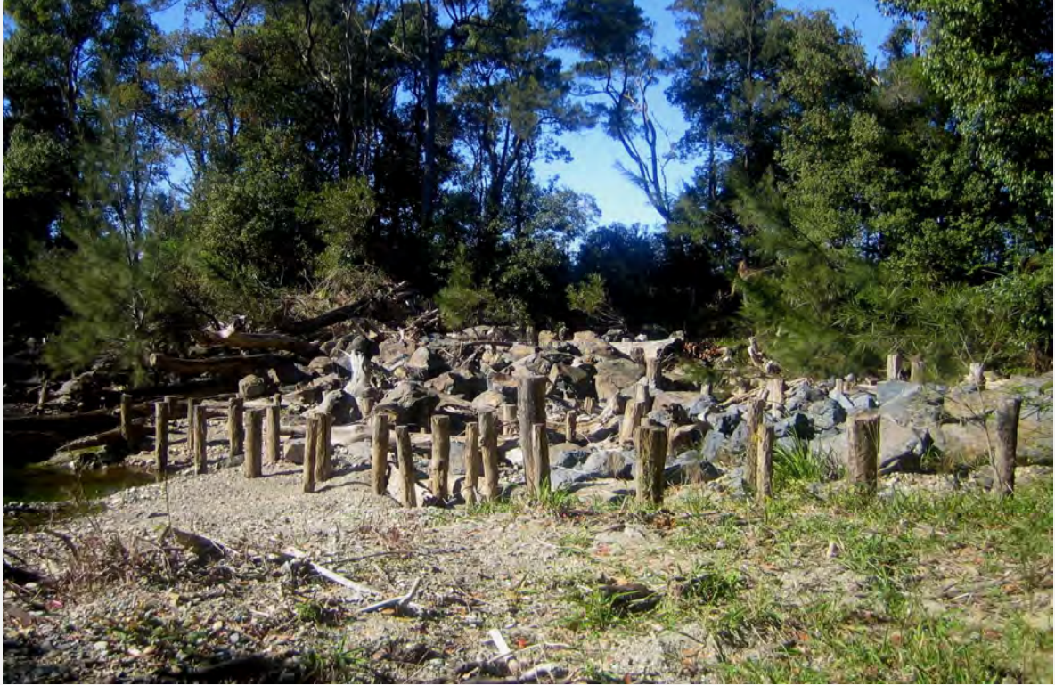
Photo below: 'Pins' Inserted on Outside Bend to Create Geomorphic Structure and Stability
